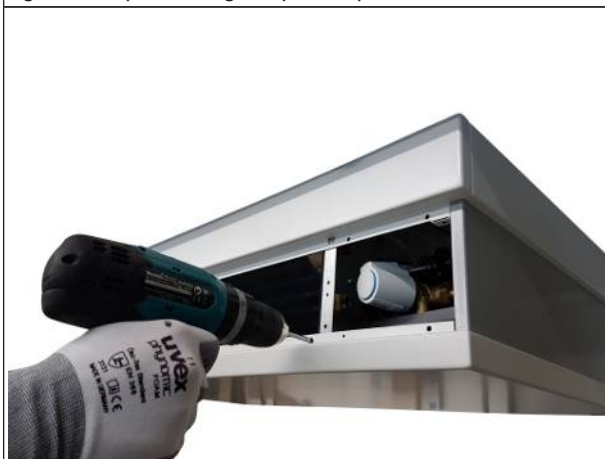
Fig. 10: Fix the casing with screws
