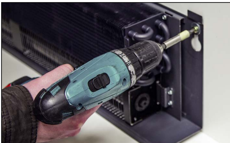
Fig. Fixing the mounting frame to the wall Fix the mounting frame to the wall on the left and right hand side.
