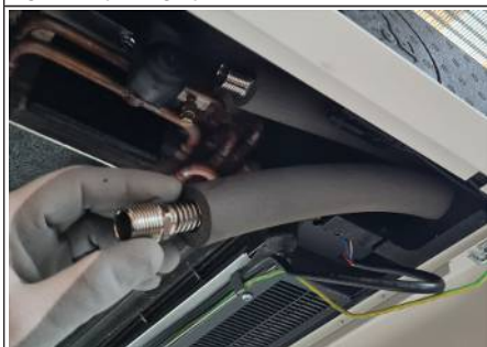
Fig. 17: Flexible corrugated pipes
