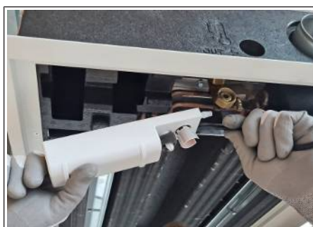
Fig. 44: Dismantling the condensate pump
