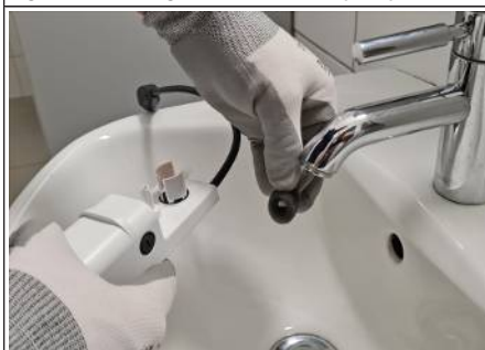
Fig. 46: Cleaning the dirt filter
