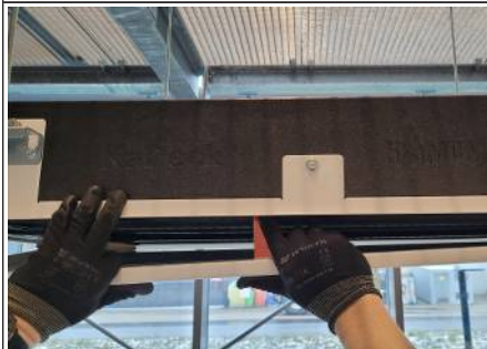
Fig. 8: Pressing in the retaining plate
