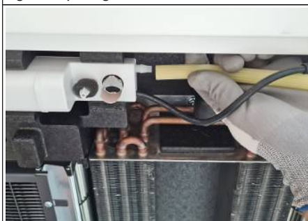
Fig. 21: Fixing the condensate hose to the condensate pump
