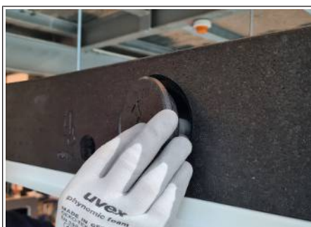
Fig. 23: Removing the primary air spigot
