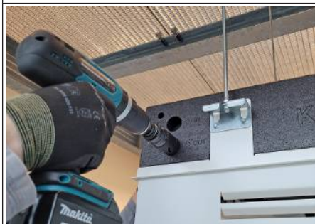
Fig. 16: Opening up the connection holes
