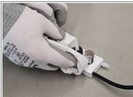
Fig. 45: Cleaning the condensate pump
